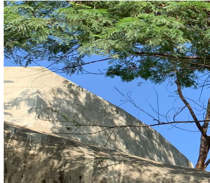
Mureta chumbada executada
